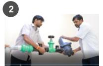
Press on the tips of the thread to make sure the tape adheres fully to the support Connect the previously sealed male end to the female end and proceed manually by screwing the two elements
