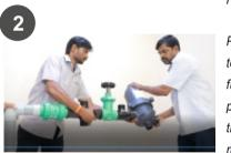
Press on the tips of the thread to make sure the tape adheres fully to the support Connect the previously sealed male end to the female end and proceed manually by screwing the two elements
