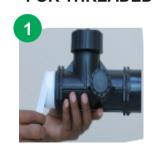
Start winding some PTFE sealing tape on the outside of the threaded male end, taking care not to obstruct the through-hole on the pipe, fitting or valve Complete the first winding layer by winding the tape clockwise until you reach the root of the thread.
